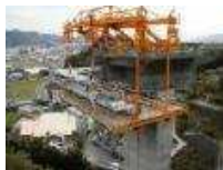
Shin-Tomei Expressway pier construction
