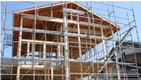
Example of construction of wedge binding type scaffolding "Shinwa Catcher" for a house.
