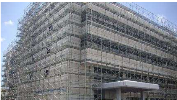
Example: Wedge binding-type scaffolding, "Shinwa Catcher," for mid-rise structures
