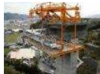
Shin-Tomei Expressway pier construction
