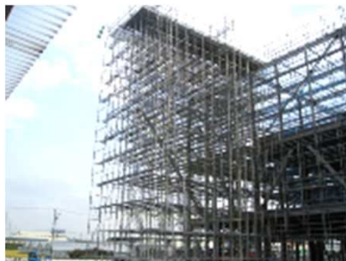
Large-scale warehouse/roof forming construction work
